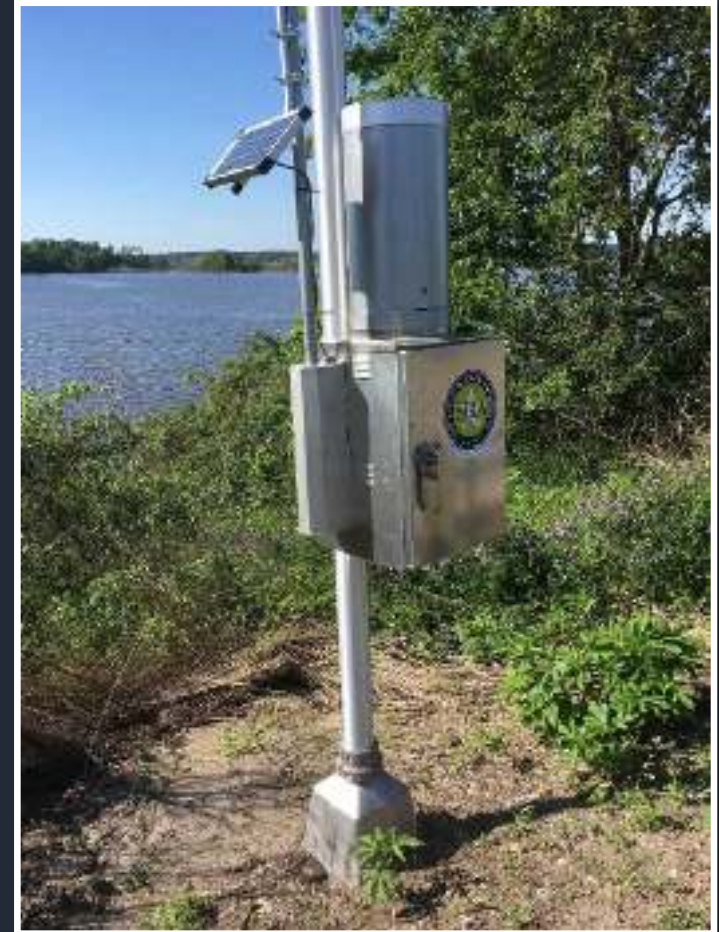
New Installation at FM 1375
